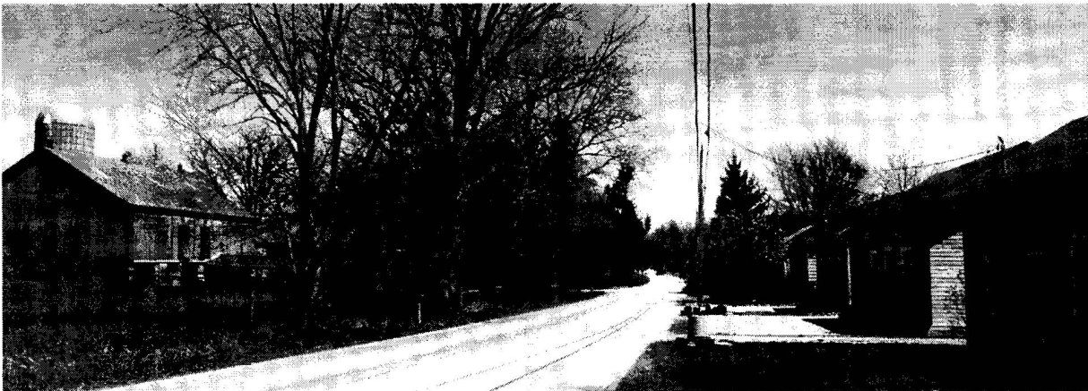
Image 13: View of Greenfield Road looking east, 2013
