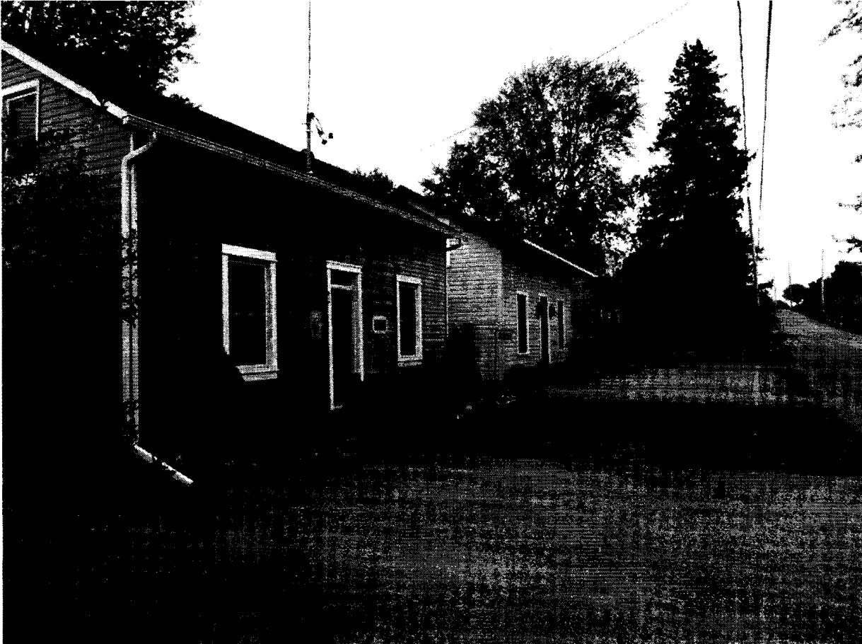
Image 16: The unified massing and setback of the worker's cottages creates a consistent visual rhythm along the road
