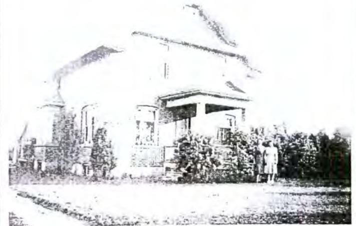
Clarence Heise house , 1945. GPA # 6A
