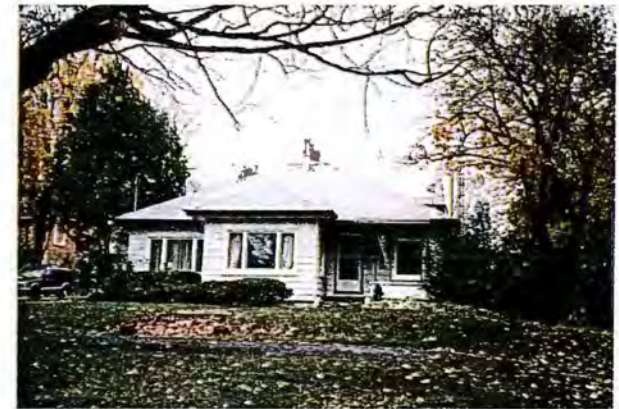
The house was still close to its original configuration in the fall of 2005.
