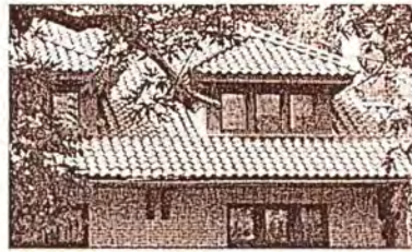
FIGURE 28: CLAY TILE ROOF
