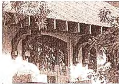
FIGURE 35: WOOD EAVES BRACKETS
