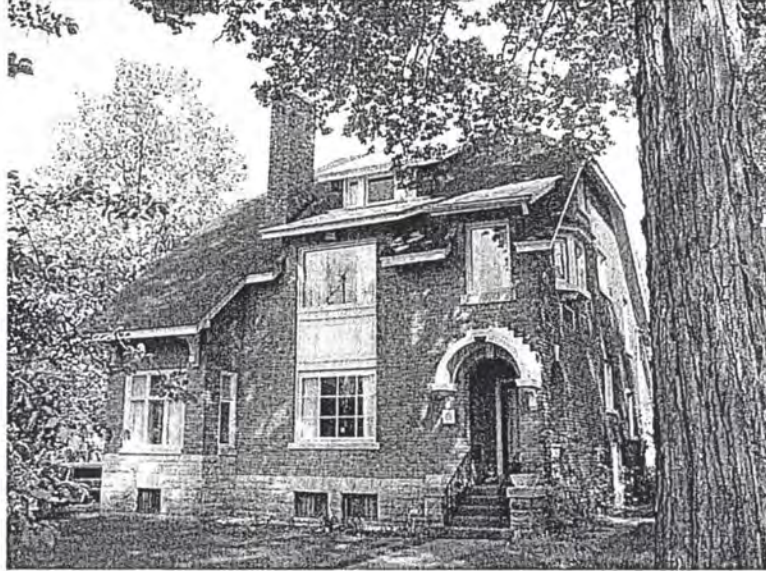
This two-storey yellow brick-clad house with a stone foundation has a rectangular floor plan and truncated hip roof with a shed dormer. This house has wide overhanging eaves and large wooden eaves brackets. The side hall plan features an arched entranceway with an arched stone hood over the front door. The house faces onto Central Park.
