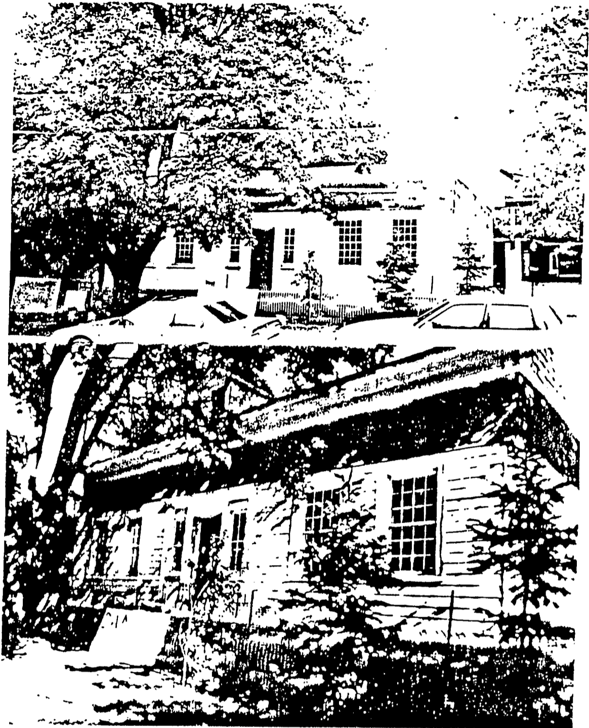
TOP AND BOTTOM: MAIN (WEST) FACADE
