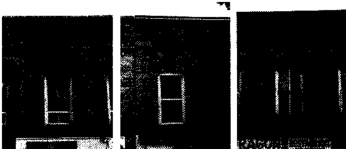
Replacement windows that lose original character of shape and glass division
