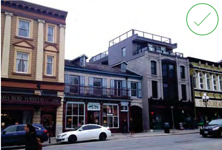
115. Rooftop addition on historic commercial building in downtown Kingston. The addition has a simple design and is set back from the front façade, which minimizes its impact on the historic building. (Source: ERA)
