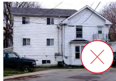
84. Incompatible side addition that visually overwhelms the principal house and does not complement the design and rhythms of the existing building (Source: ERA)
