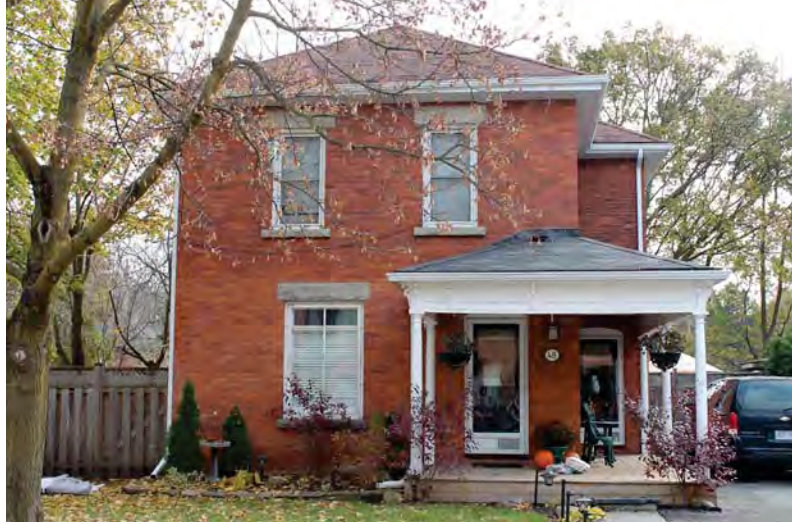
195. Contributing Building at 48 Sterne Street, Bolton. (Source: ERA)
