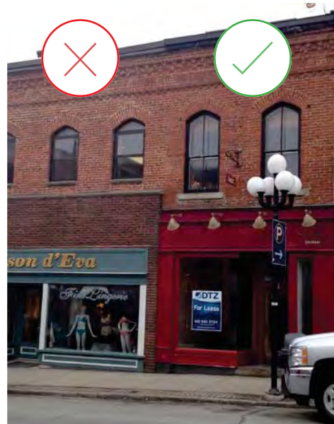
103. Note the difference between conserved historic windows on the right and the modern replacements on the left. The new storefront on the left does not take into consideration the original window glazing pattern and proportions and as a result the new windows are not compatible with the architectural style of the building, Kingston, Ontario. (Source: ERA)
