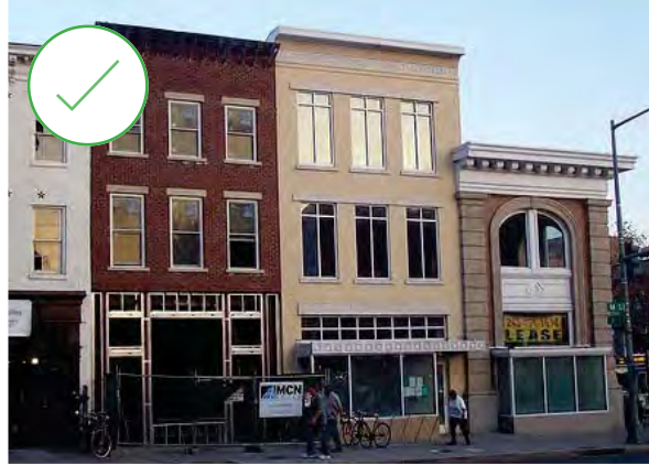
119. New infill is compatible in height and design with adjacent historic buildings, Washington, DC. (Source: Richard Layman, Flickr).
