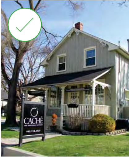
127. A ground sign and hanging sign do not conceal the building's architectural detailing, Kleinburg-Nashville HCD. (Source: ERA)
