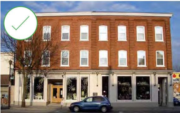
120. Left hand side of building was re-built following fire damage, Picton Main Street HCD. (Source: ERA)
