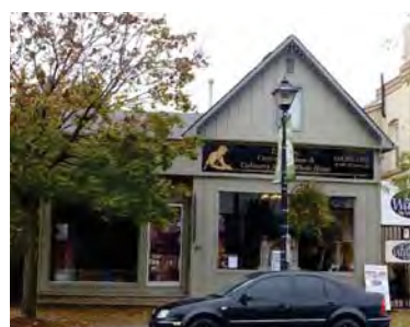
126. Pitched roof at 46 Queen Street North, Bolton. (Source: ERA)
