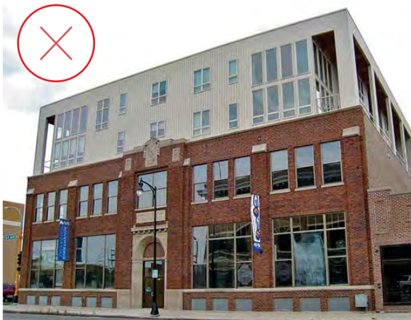
117. Rooftop addition that overwhelms the scale of the existing building. (Source: National Park Service, U.S.)
