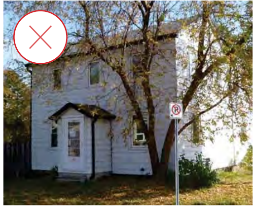
43. The size, proportions and texture of vinyl and aluminium siding are incompatible with the style of historic buildings in the District, 26 Mill Street (Source: ERA)
