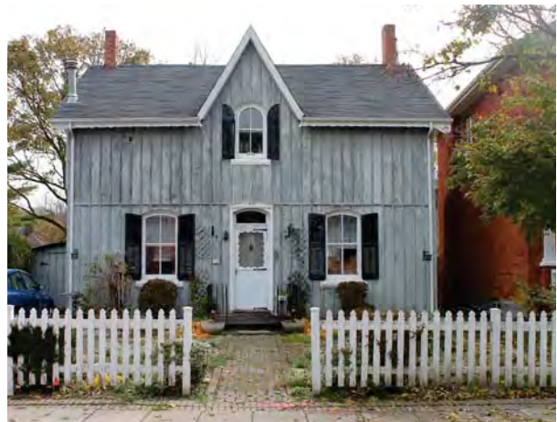
38. Wood picket fencing at 52 Sterne Street, Bolton. (Source: ERA)
