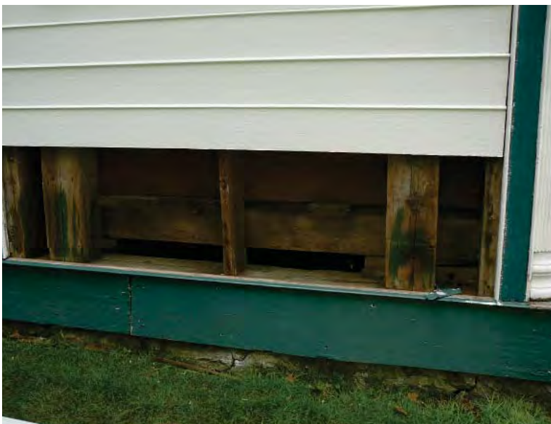
55. Investigate and document existing conditions and construction before repairing and replacing cladding. (Source: ERA)
