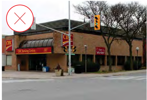
123. Unsympathetic post-war single storey bank building at 2 King Street East, Bolton. (Source: ERA)
