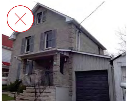
45. Grey brick cladding conceals original masonry and architectural detailing on this historic house in Kingston, Ontario (Source: ERA) (Source: ERA)
