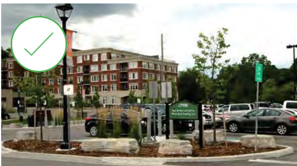
141. Refreshed and improved Ann and Samuel Sterne Municipal Parking Lot, Timothy and Ann streets, Bolton. (Source: Town of Caledon)
