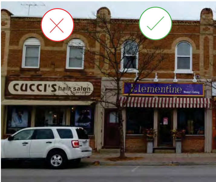
102. Original window openings and patterning have been maintained in new window design and installation at 19 Queen Street North (right) in contrast to poorly modified window openings on 23 Queen Street North (left), Bolton. (Source: ERA)
