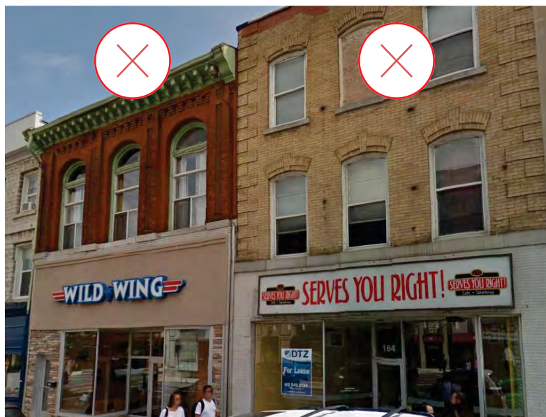
113. The signage on the left is inappropriately proportioned, obscuring architectural detailing on the historic building. The signage on the right is correctly located but the box design with internal lighting is not compatible with the architectural style of the building or the character of the streetscape, downtown Kingston. (Source: Google)
