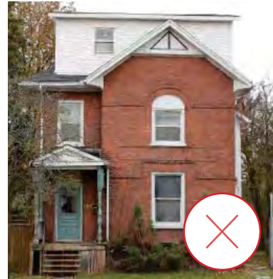
83. Incompatible rooftop addition that disregards the original roof shape and architectural style of the house. (Source: ERA)
