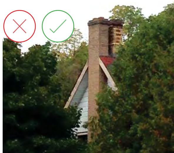
Re-roofing of original chimney. 11 N. ... R
