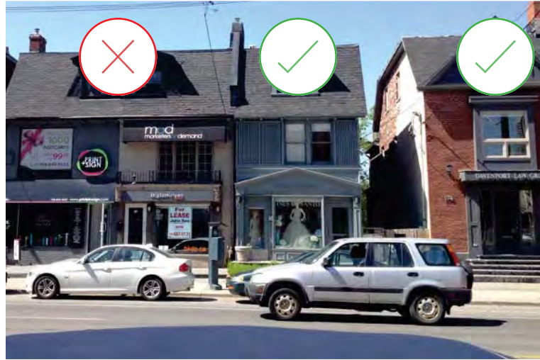
128. Several different design approaches to commercial conversions along Davenport Road, Toronto, all of which retain the residential character of the buildings. (Source: ERA)
