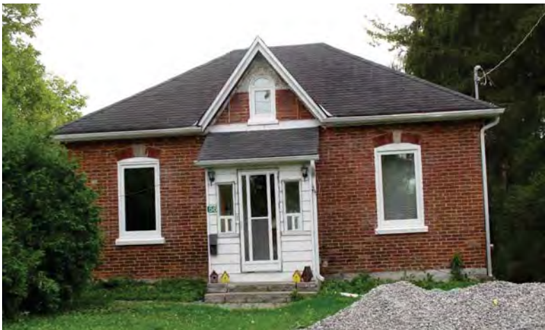
50. The removal of synthetic siding at 56 Nancy Street revealed the original brickwork and architectural detailing, Bolton. (Source: ERA)
