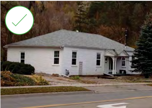
44. Original or traditional horizontal board cladding at 97 King Street East, Bolton. (Source: ERA)
