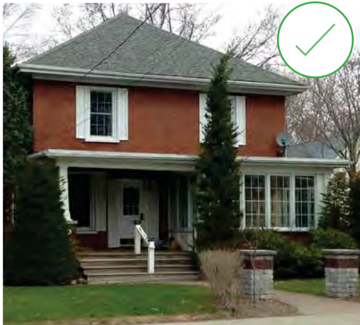
77. This porch enclosure respects the proportions of existing house and retains original porch elements such as the columns. Bloomfield, Ontario. (Source: ERA)
