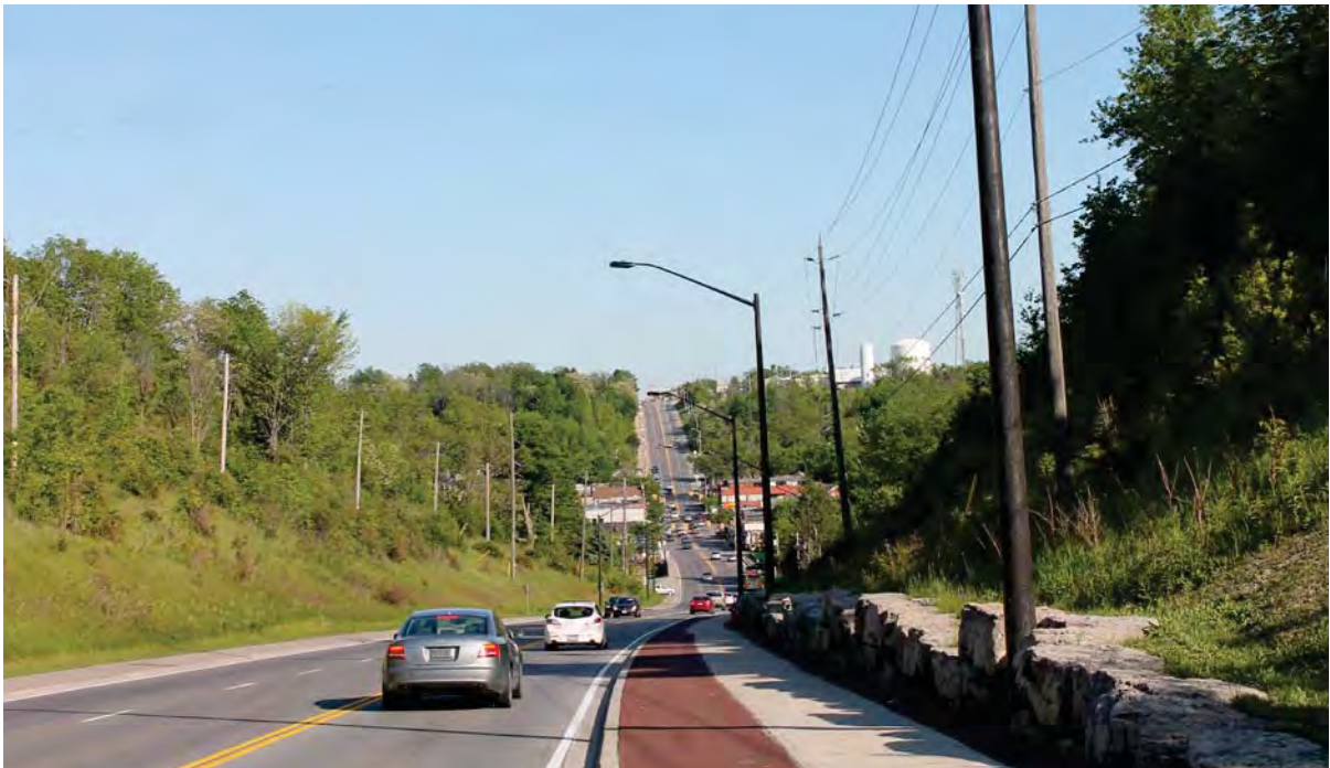
181. Looking south along Queen Street from top of north hill, Bolton. (Source: ERA)
