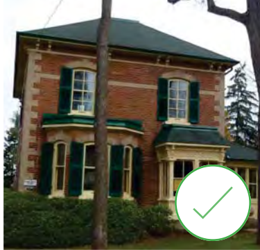
63. Historic shutters at 31 Nancy Street, Bolton. (Source: ERA)
