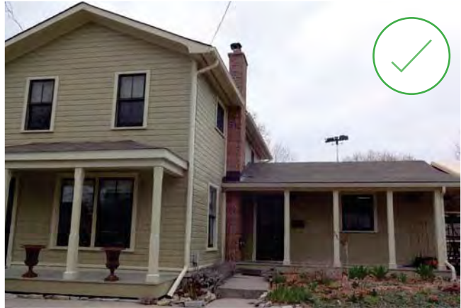
76. Compatible new porches on both principal house and addition, Barriefield HCD, Kingston, Ontario. (Source: ERA)
