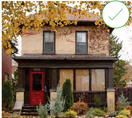
78. The enclosure of this historic porch maintains existing horizontal and vertical rhythms as well as architectural elements of this Edwardian Classical house in Peterborough, Ontario. (Source: ERA)
