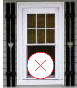
64. Inappropriately proportioned new shutters. (Source: www.oldhouseguy.com)
