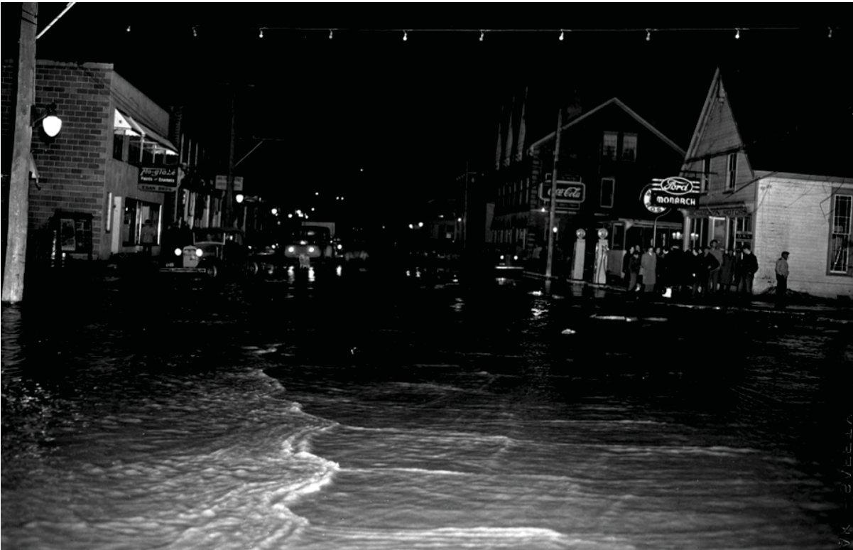
167. Bolton flood, looking south along Queen Street North near Mill Street, 1950. (Source: courtesy of PAMA)
