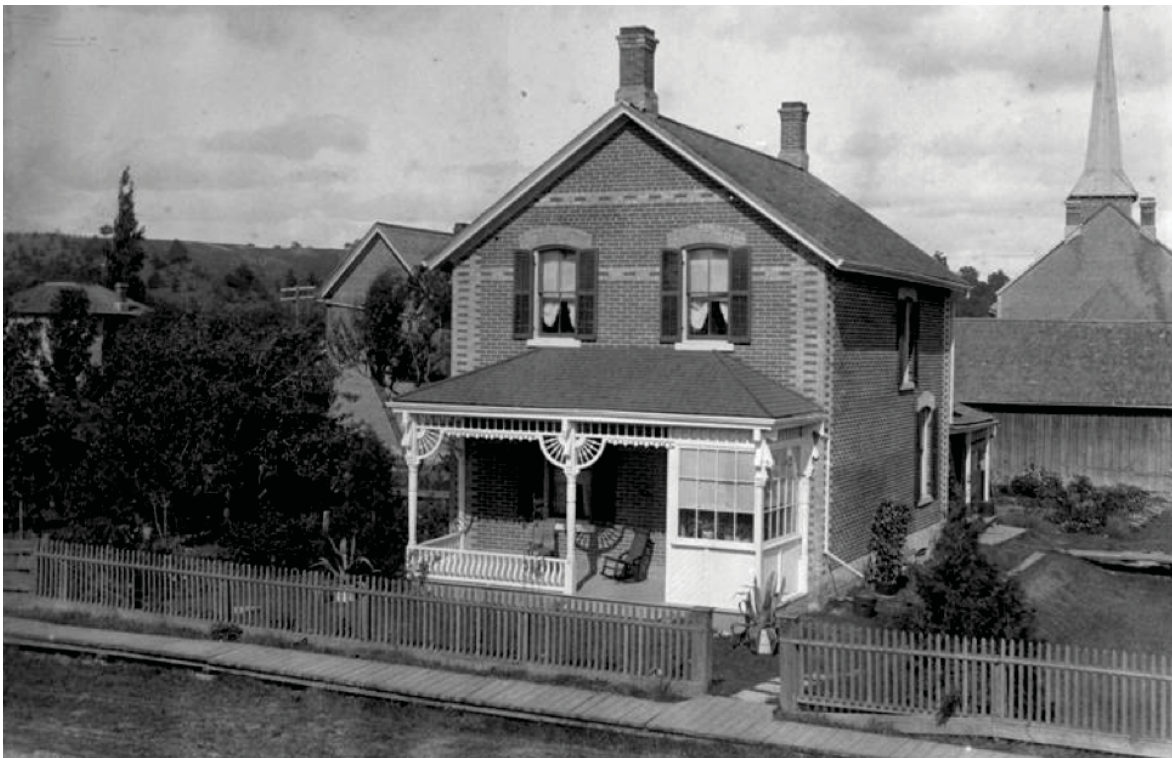
96. Rectory for Christ Church Anglican, 11 Jane Street, Bolton. (Source: courtesy of PAMA)
