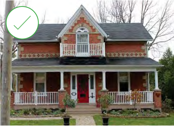
42. Decorative brickwork featuring orange-red coloured brick, which is common in Bolton, 38 Nancy Street. (Source: ERA)
