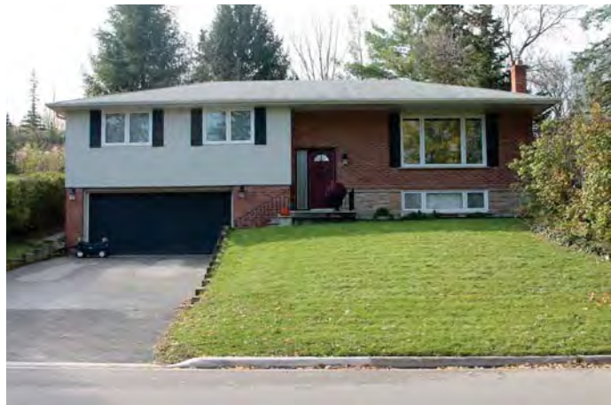
14. Non-contributing property in the Village of Bolton HCD, 26 Jane Street. (Source: ERA)
