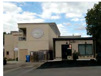
135. Improved rear elevation of 52-56 Queen Street North facing the Ann and Samuel Sterne municipal parking lot and Timothy Street, Bolton. (Source: Town of Caledon)
