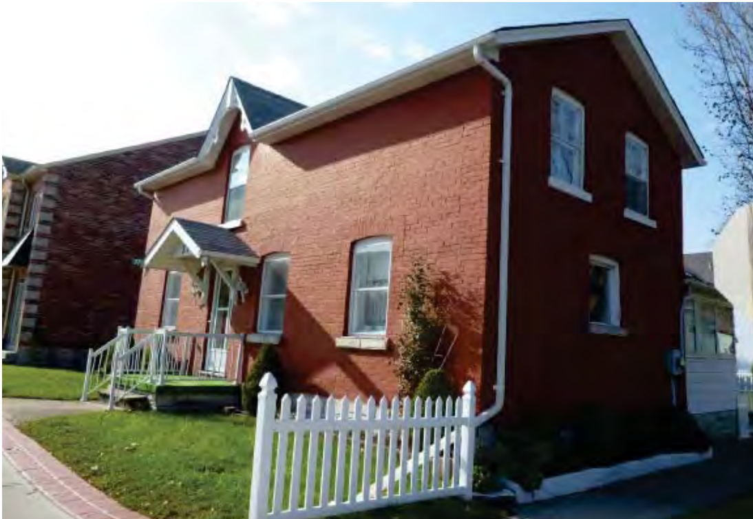
204. 37 King Street East, 2013. (Source: ERA)
