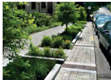
161. Tree planting pits can act as infiltration rain gardens during flooding events, Portland, Oregon. (Source: City of Portland)
