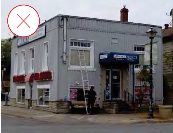
100. Original architectural detailing is concealed by modern metal cladding on 40 Queen Street North. In contrast to parging or stucco, this cladding could be more easily removed to reveal original cladding, design and detailing. (Source: ERA)
