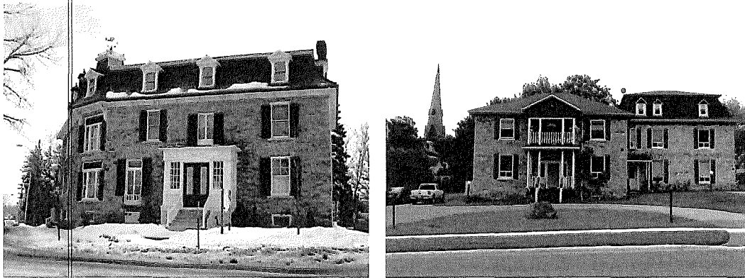
Figures 24 – 25: left – Beaver Hall Bed and Breakfast, 75 King St. W., Gananoque (photo E. Tumak, Jan. 2008); right – 181 King St. W., Gananoque—the wing at the right/west is a later addition (photo E. Tumak, July 2009). Note both are constructed of sandstone.
