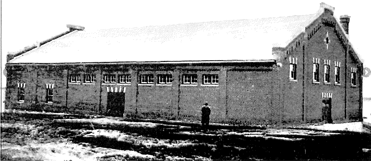
Figure: 1000 Islands Playhouse, Firehall Theatre, viewed from the northwest shortly after construction ca. 1912, showing the detailing of the west gable ( http://www.1000islandsplayhouse.com/firehall-theatre/ , accessed Sept. 2019, no attribution provided for original source).
