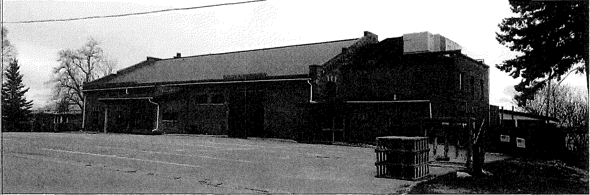
Figure: 1000 Islands Playhouse (former Drill Hall, then Firehall and Police Station), 185 South Street, viewed from the northwest, showing a later addition to the right/west (E. Tumak, May 2020).
