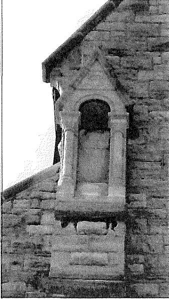
Figure 20: Detail of niche atop front façade buttress (E. Tumak, Jan. 2020).
