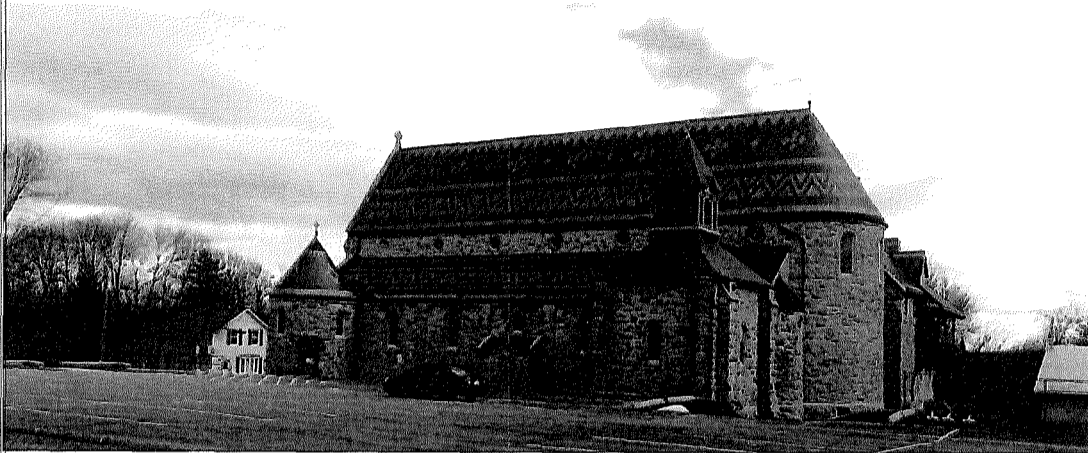
Figure 23: North elevation of St. John's viewed from the northwest (E. Tumak, March 2020).
