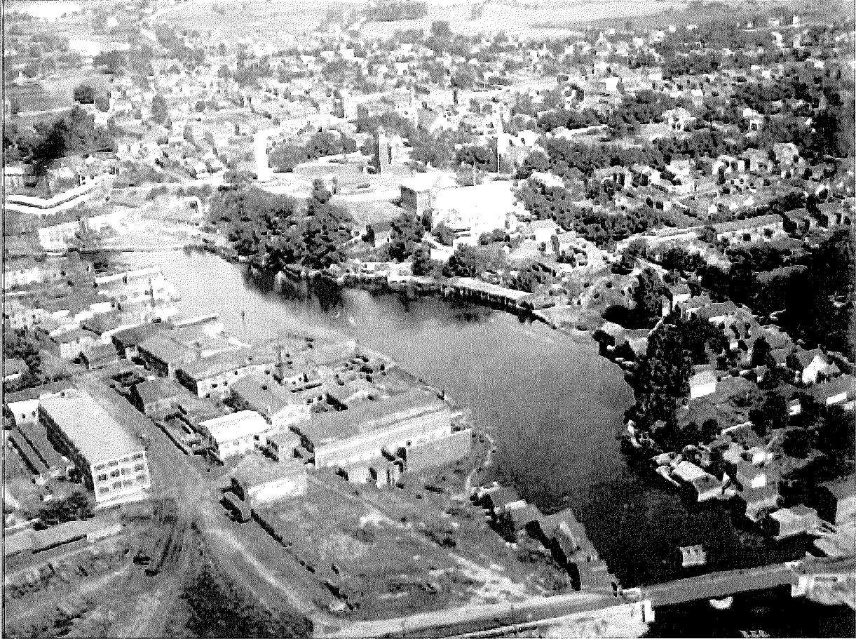
Figure 39: Oblique aerial, 1920, from the southwest, with St. John's visible roughly in the centre left of the image (McCarthy, LAC MIKAN no. 3261445).
