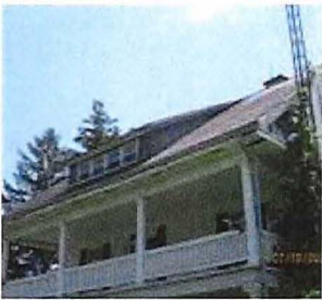
2. Steeply pitched side gable roof with slate cladding, shed roof dormer, two brick chimneys, and concrete chimney.
