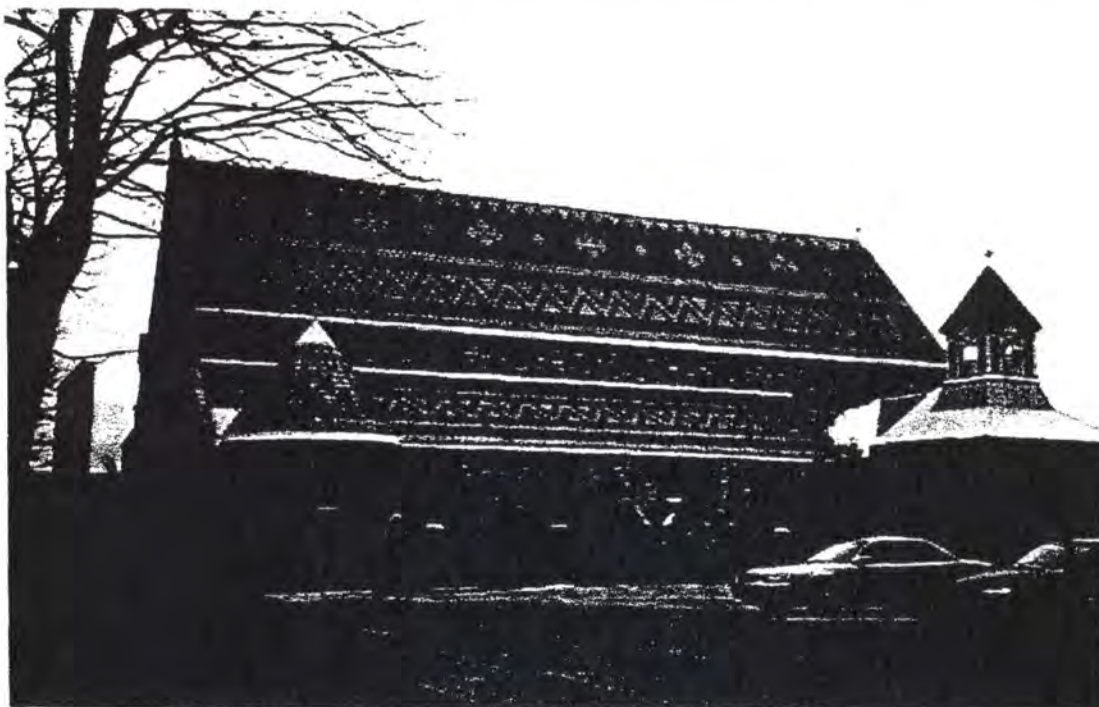
Fig.1: North elevation, particularly fine patterned dichromatic slating.
