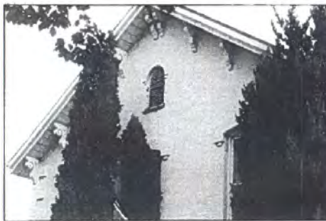
Original brackets on front façade
