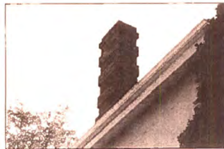
Unusual heavy banded brick chimneys (two)
