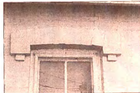
Less elaborate voussoirs on secondary windows
