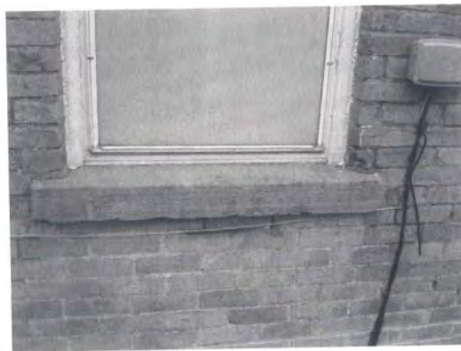
Cut stone sills and thresholds with decorative texturing
