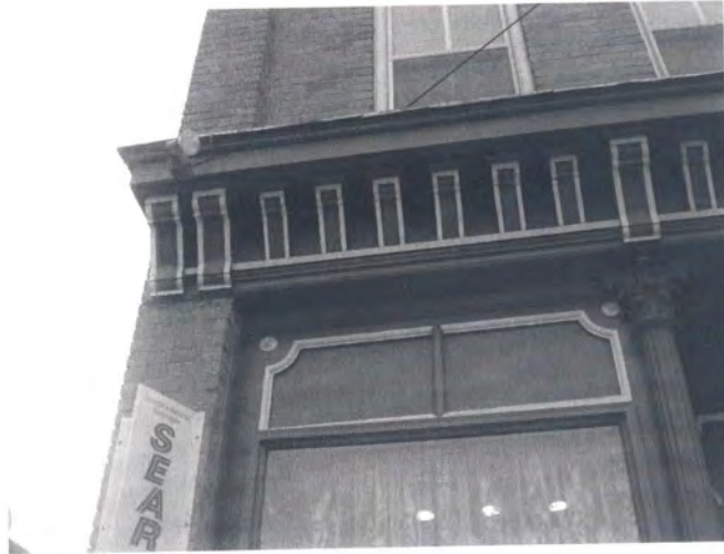
Upper window glazing, brackets, and heavy moulded cornice
