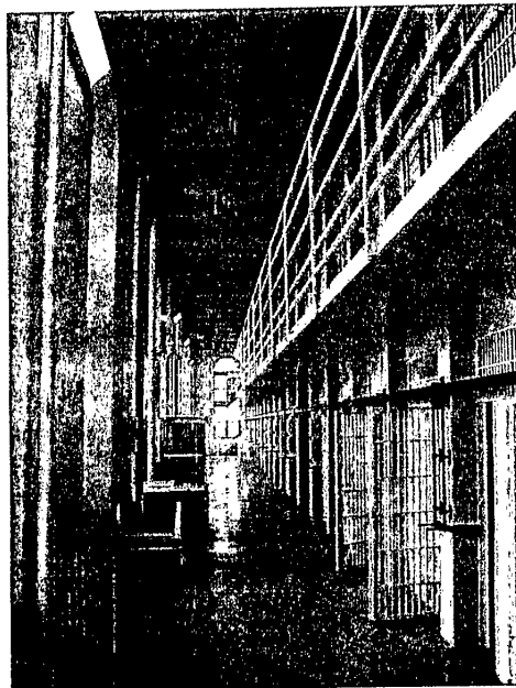
Figure 4: C-16 (Cellblock) Building – Southern Range (2005)
