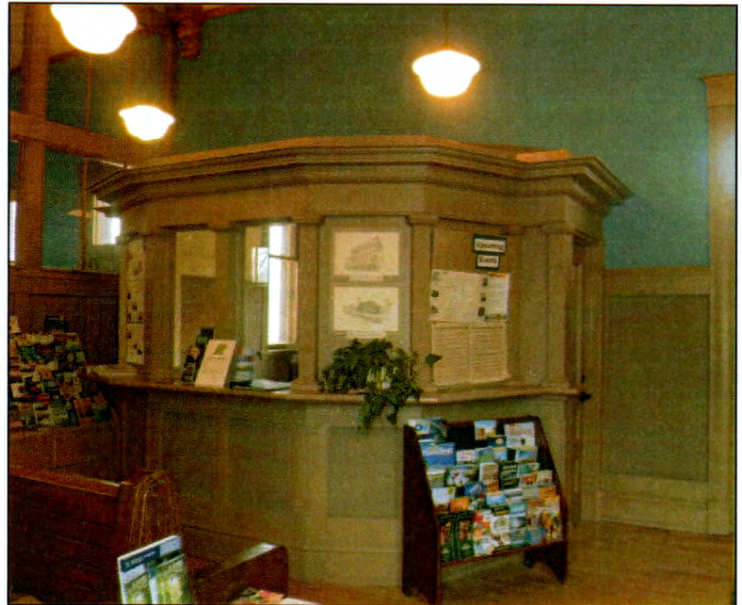
Operator's bay, projecting into the waiting area with windows and counter in place; door to office on right.
