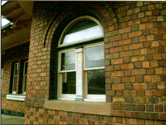
A view of the east-facing window complex showing lintel, semi-circular light above two double-hung windows with bracket between.
