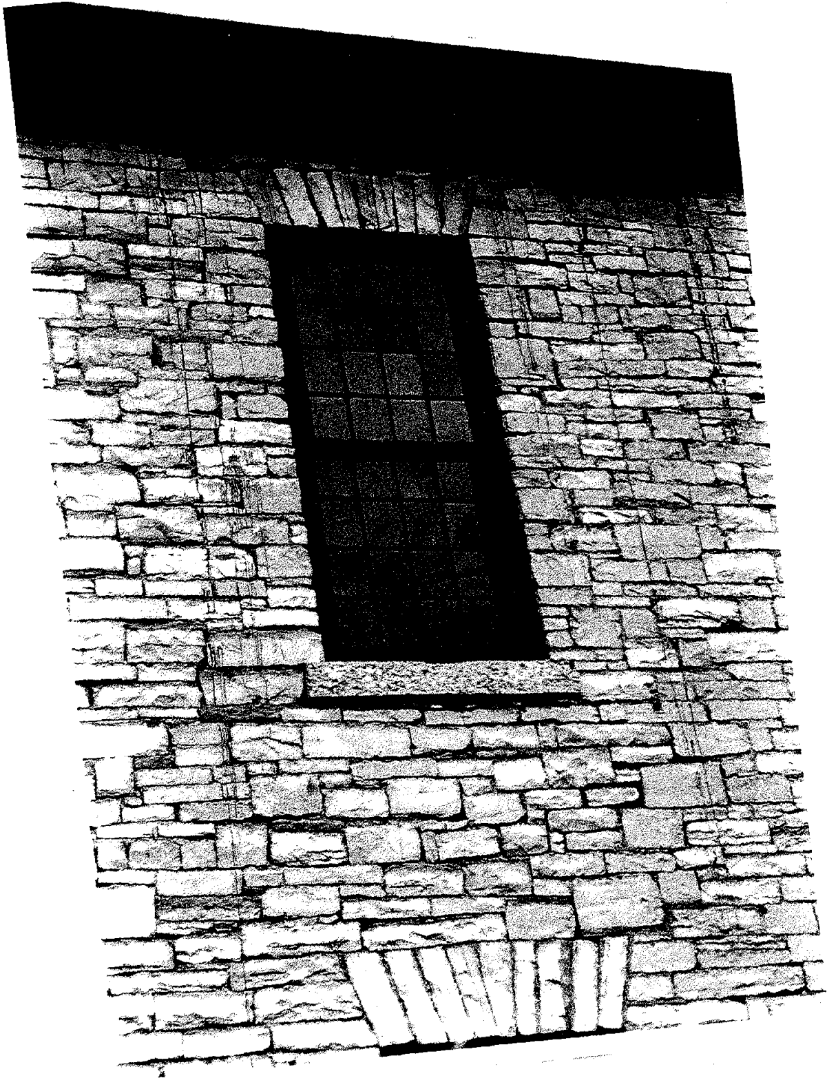
Detail view showing second storey window of warehouse portion of the Mississippi Textile Mill. .../D12
